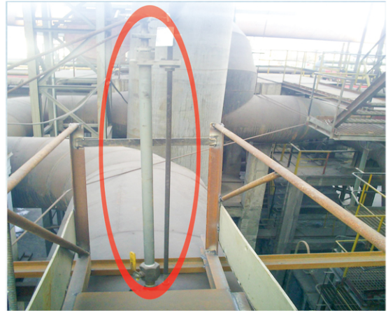
Product: BF10 Velocity-Averaging Tube Flow Sensor
